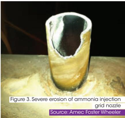
Figure 3. Severe erosion of ammonia injection grid nozzle
