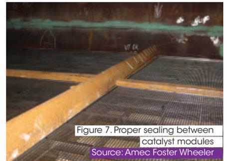
Figure 7. Proper sealing between catalyst modules
