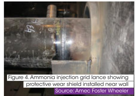
Figure 4. Ammonia injection grid lance showing protective wear shield installed near wall
